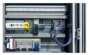
Control cabinet of the LED lighting system with the CX5020 Embedded PC (bottom) and the associated EtherCAT Terminals.
