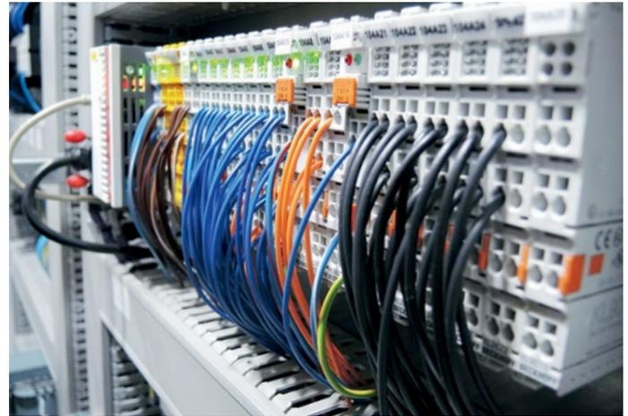
The modularity of the Beckhoff terminal system allows subsequent changes and additions at any time and little cost.
