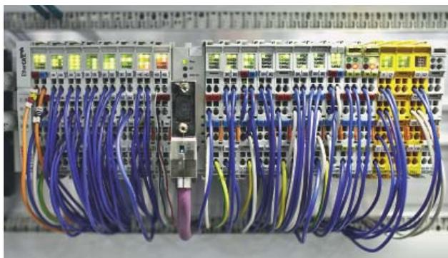
All the safety devices in the line, together with all the emergency stop buttons along the transfer route, are operated via the TwinSAFE terminals integrated into the Beckhoff I/O system.
