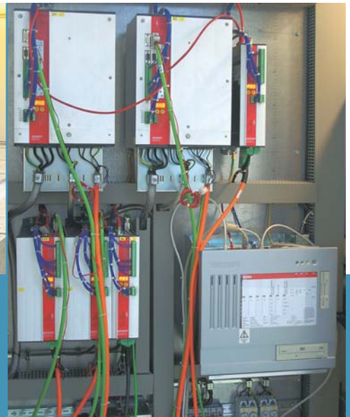
AX2xxx Servo Drives for controlling highly dynamic linear motors
